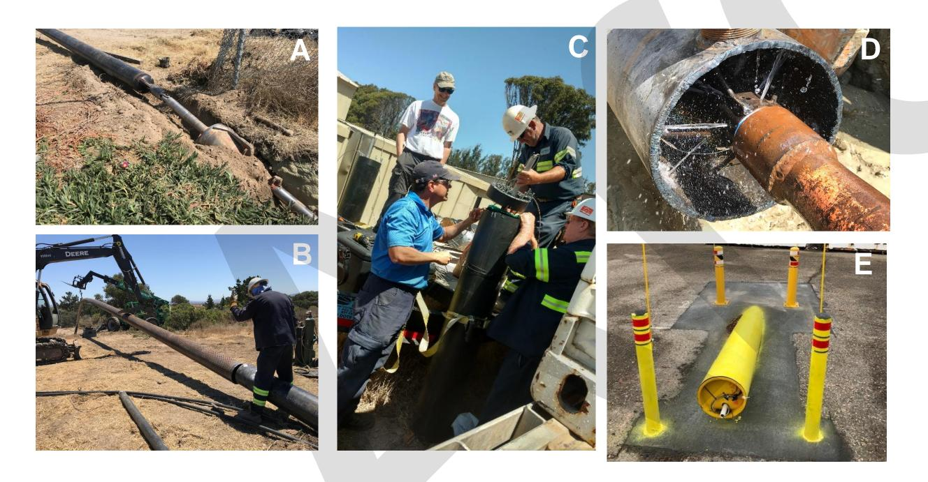
**Figure 7.** A: Reaming the borehole with 18-inch reamer. B: Aligning screen section prior to welding. C: Final construction of the PVP monitoring cartridge. D: Jetting tool for well development. E: Wellhead completion.
