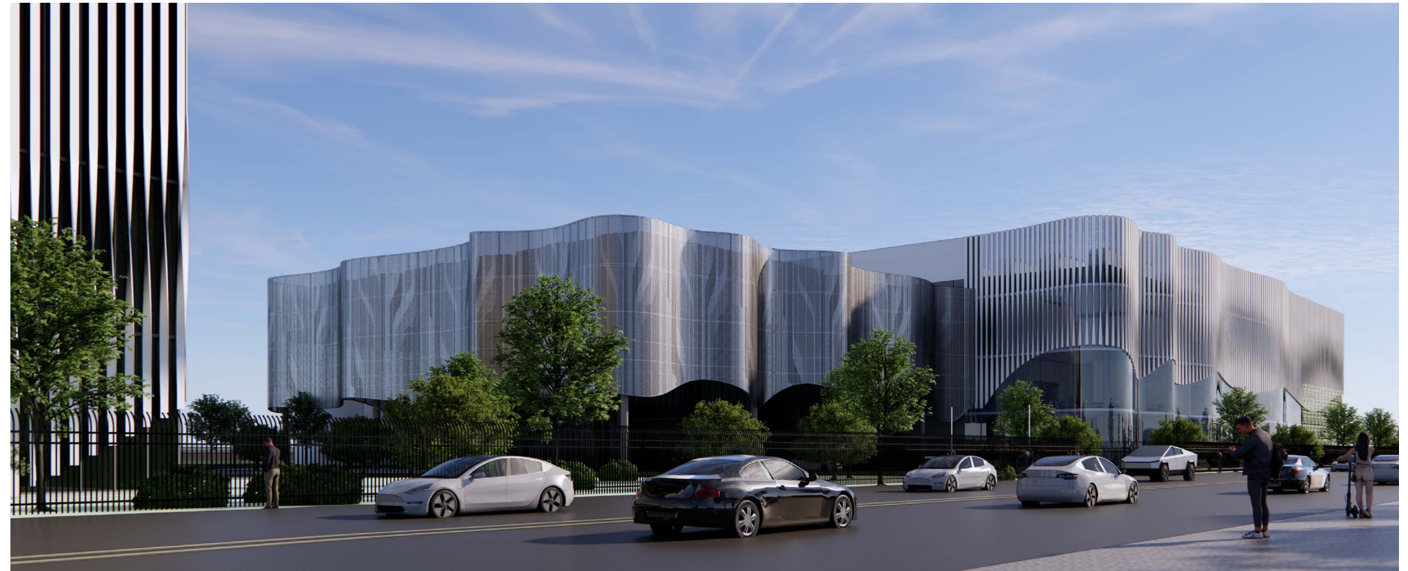
Terra Data Center, San José, California, USA
